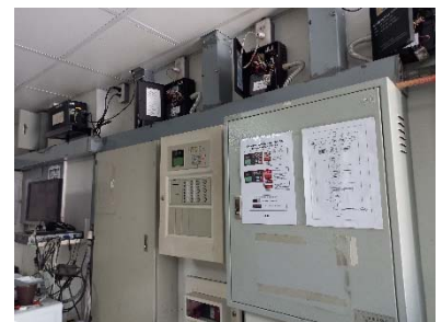
Fire Fighter Telephone System
